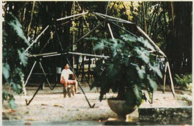
**FIGURA 3. DOMO GEODÉSICO COM PEÇAS DE BAMBU E CONEXÕES DE METAL, DESMONTÁVEL E COM PESO TOTAL EM TORNO DE 70 KG, ARMADO EM ÁREA DA PRÓPRIA UNIVERSIDADE.**
